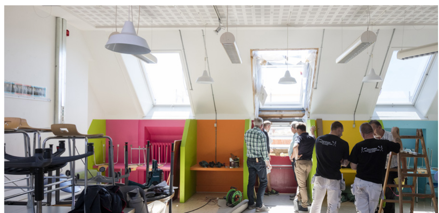
Installation phase of the roof windows
